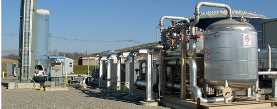
Figure 7. Example of a Venture Engineering Gas Conditioning Skid
